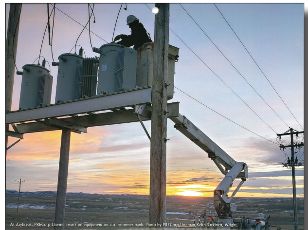
At daybreak, PRECorp Linemen work on equipment on a transformer bank. Photo by PRECorp Lineman Keith Salkmen, Wright.
