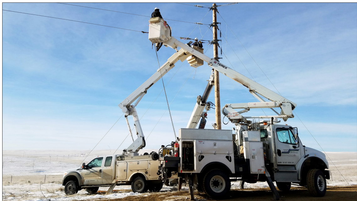
The PRECorp Line Crew from Wright works on an overhead power line.
